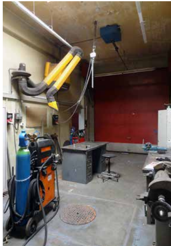
Un garage (photo Y. Delemontey, 2019).
